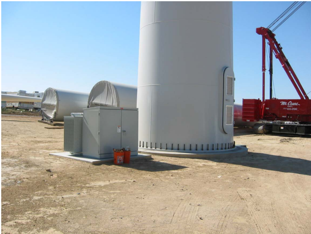
Figure 6-1. Typical Wind Turbine Transformer Arrangement.
