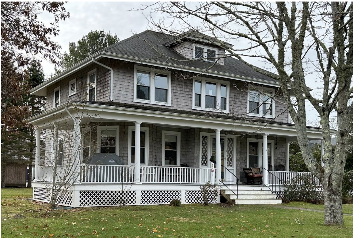
Photo 2. View from Cottage Street, looking southwest.
